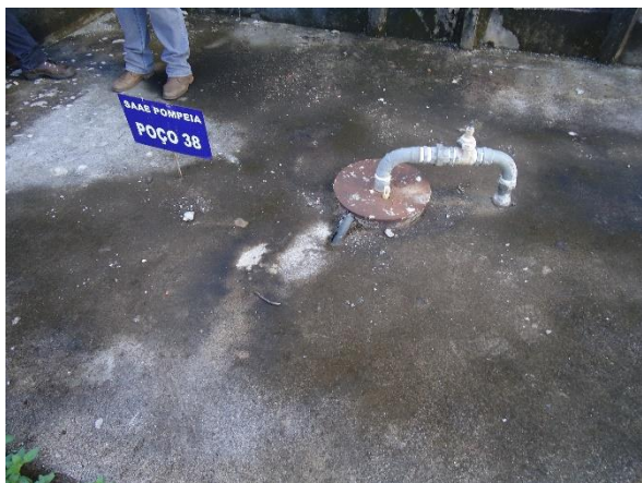
Foto 3.25 – Poço 38 – Dist. Industrial III
