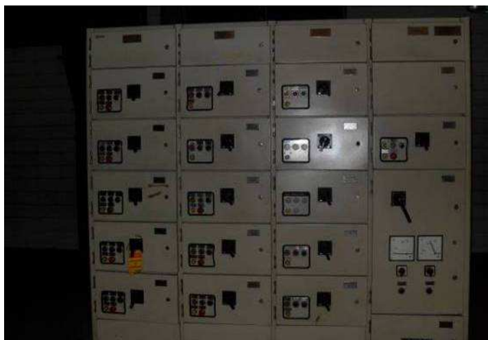
Figura 166 - Painel do CCM – 460 V
