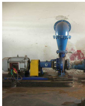
Unidades de recalque: 1x75CV + 2 x 50 CV (planilha ref. 1), ou 1 x 70CV + 1 x 50CV + 1 x 40CV (planilha ref. 2)
